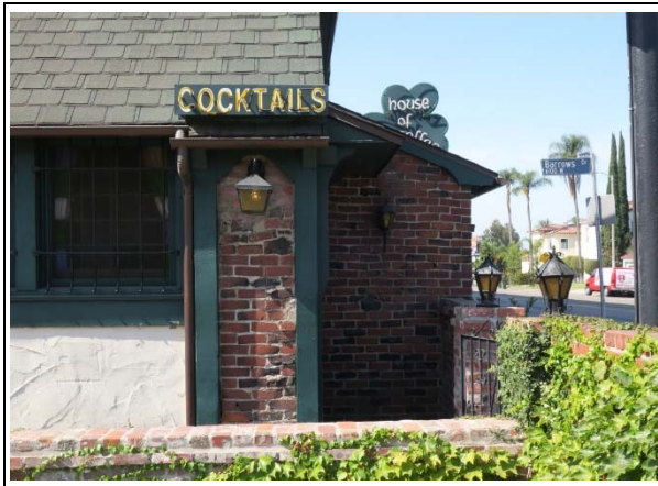
Detail of textured stucco and clinker brick wall cladding on north façade (ARG, 2018)
